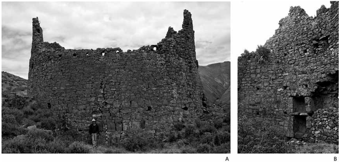
Figure 7. Exterior (a) and detail of interior (b) of circular structure at Karway, northern Conchucos. It resembles D-shaped structures: imposing height, unroofed interior space, inward leaning walls. The buildings feature a series of double niches that may have contained funerary bundles and other cult objects. Note also the holes for rafters to support additional floors and construction.
